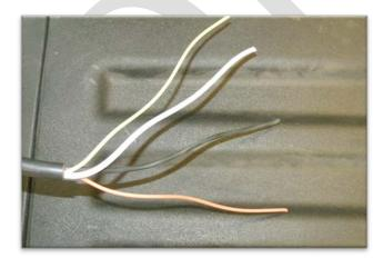
STEP 14 Cut the jacketed portion off of the conductor about 8 inches.
